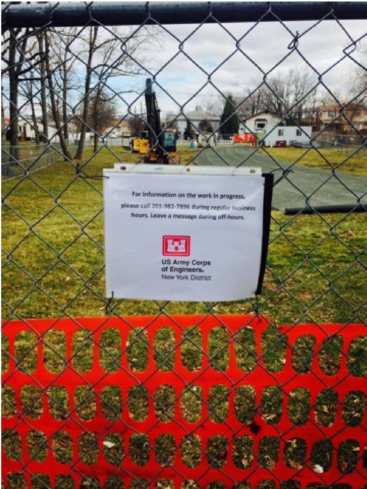
Fig. 4. Public information posting at Redstone Park Phase 1 job site.
